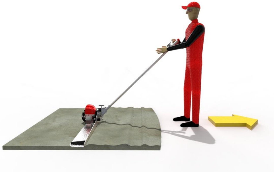
Fig. 10: worksituation during smoothing and compacting the concrete floor
